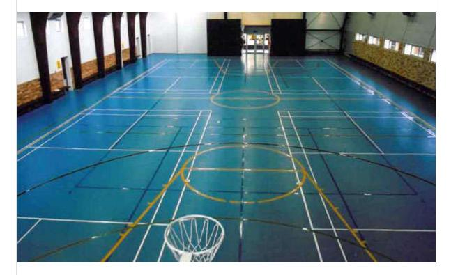
Multi-purpose Point Elastic sports flooring consisting of two layers of natural and synthetic rubber and an elastic foam supporting underlay. The calendered and vulcanised layers are joined during the production and form Mondoflex II.
