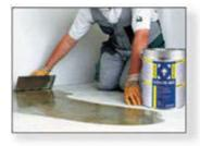
Immediately apply an even coat of the UZIN PE 480 using a B1 notched trowel.
